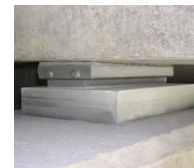
Linear rocker bearing
