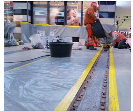
Metal expansion joints
