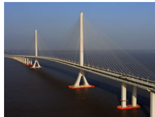
Chongming bridge, China
