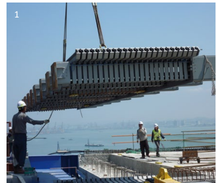
Sliding finger joint
