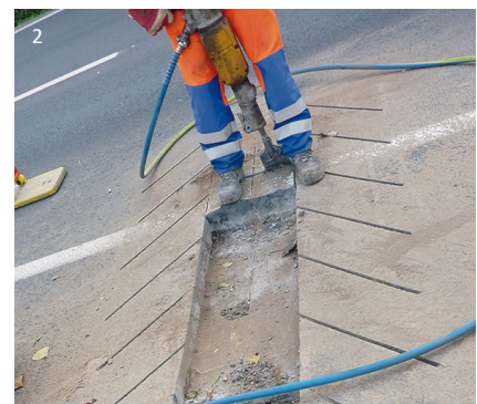
Flexible plug joint
