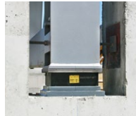
Reinforced elastomeric bearings
