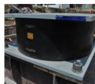
Lead rubber bearings
