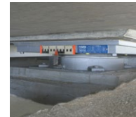
Linear rocker bearing
