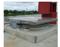
Incremental launch (ILM) bearing
