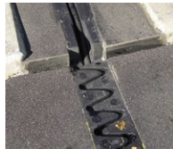
Cantilever finger joint
