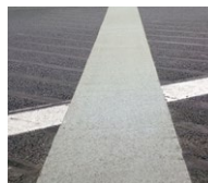
Flexible plug joint
