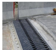
Flexible plug joint
