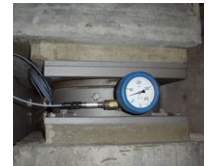
Incremental launch (ILM) bearing
