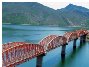
Infiernillo bridge, Mexico
