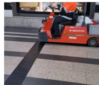
Flexible plug expansion joints
