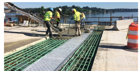
Pouring the concrete into the recess
