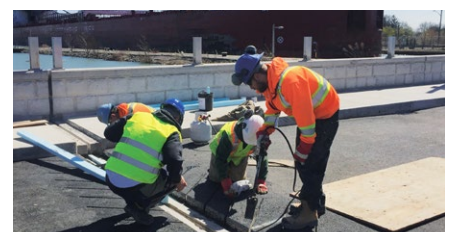
Installation of the POLYFLEX®ADVANCED PA30 expansion joint and support ribs
