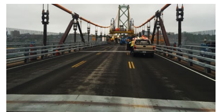
Temporary plates at the point of future installation of the expansion joints
