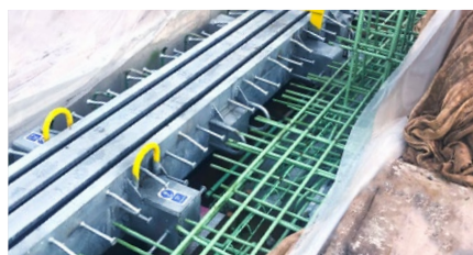
TENSA®MODULAR LR3 joint is being installed
