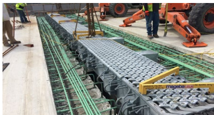
TENSA®MODULAR expansion (LR8) equipped with sinus plate noise reduction surface
