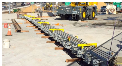
Modular joint after lifting to its final position
