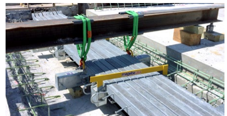
Modular joint installation
