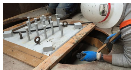
Installation of RESTON®PENDULUM Mono on terminal superstructure
