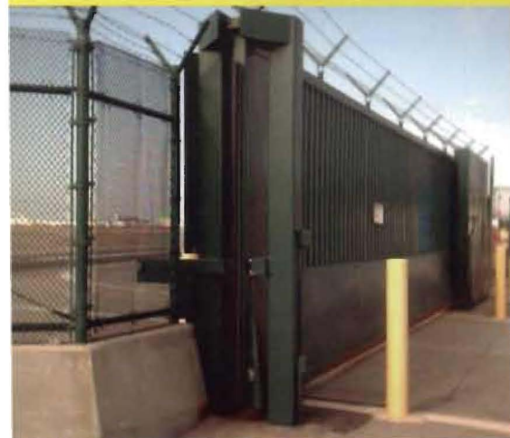
Above: Sliding Bar Gate at LAX International Airport in Los Angeles, CA. EPD sliding/crash resistant gate provides protection for active runways at International Airports. EPD gates need to be designed to accommodate various requirements including the size, speed, and type of traffic, style of the facility walls, impact and attack resistance, the need for a barrier to stop traffic, and control needs such as key pads, vehicular ID, or card reader.
