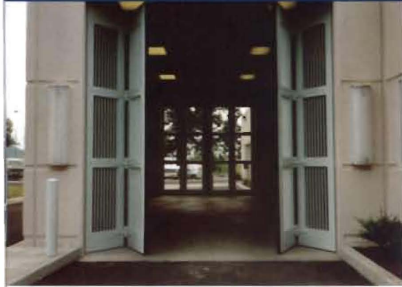
Left: EPD is a primary supplier of High Security Sally Port Doors in the United States. This is one is on the Multnomah County Inverness Jail.
