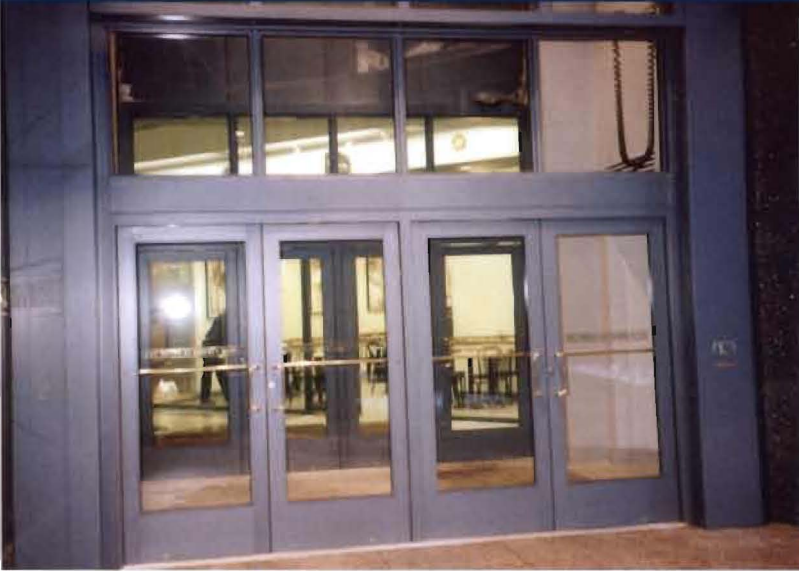
Glazed Vertical Lift Door with man doors on Liberty Place in Philadelphia, PA.
