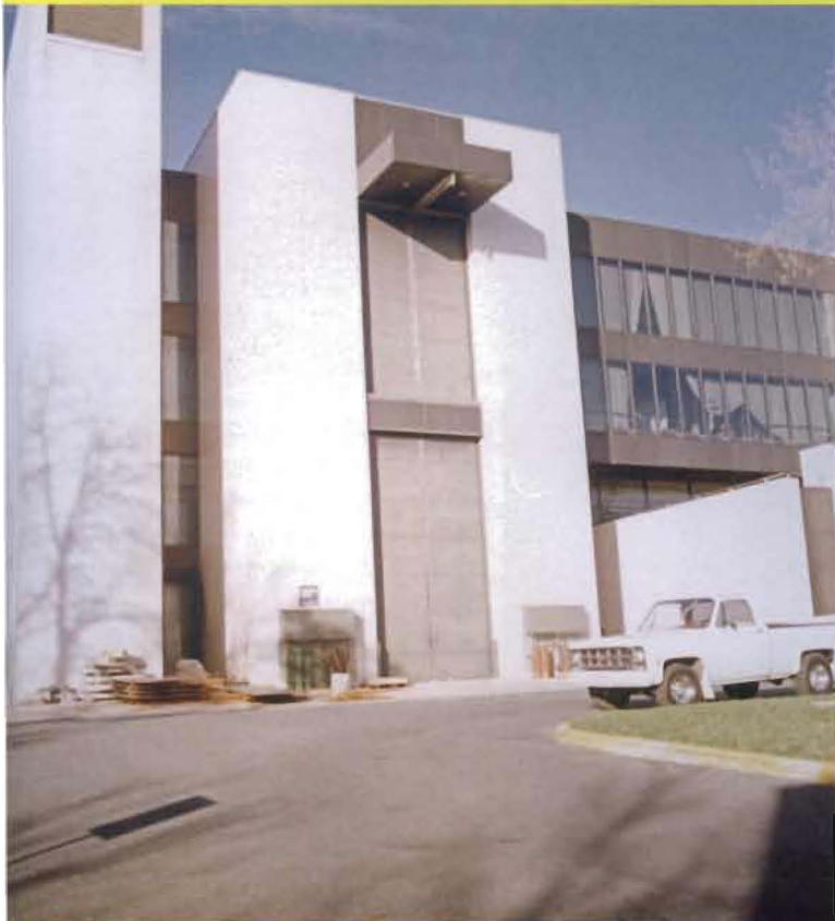
Left: This Sliding Door includes a monorail configuration. It is installed on the Performing Arts Center at the University of MN in Minneapolis, MN.
