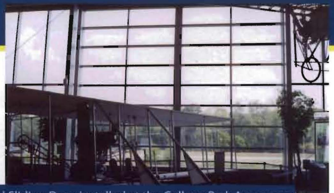
Fully Glazed Sliding Door installed at the College Park Aerospace Museum in Maryland. Sliding doors can be designed with a variety of special cladding and can include vision lights, louvers, and pass doors.
