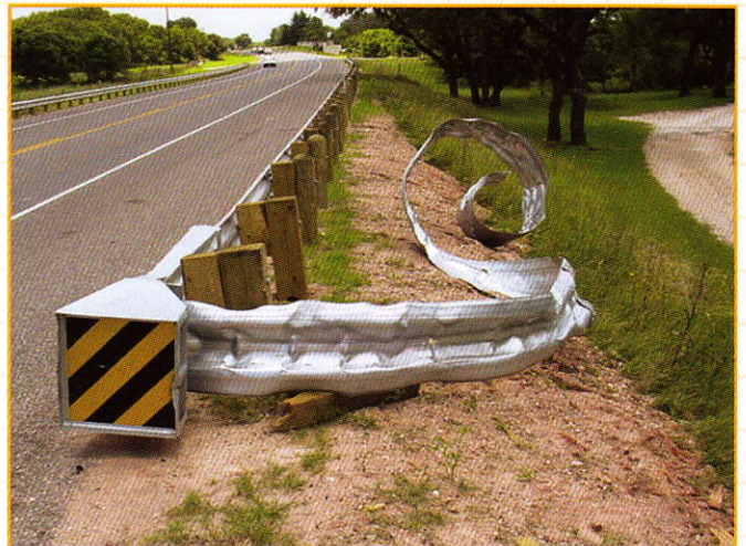
Kinetic Energy is absorbed during end-on impacts.
