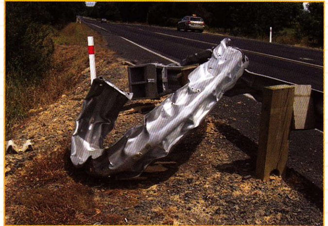
Kinetic Energy is absorbed during end-on impacts.
