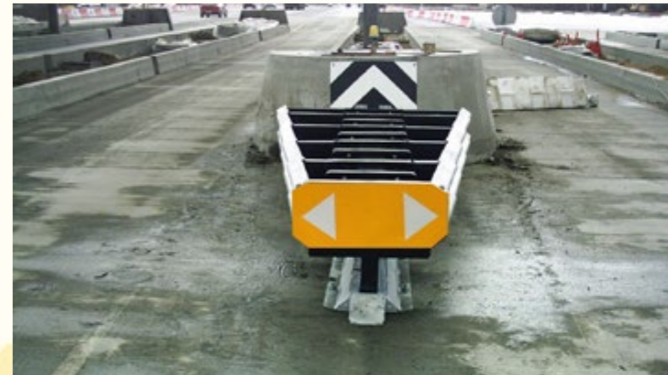
SMA 80/1 Wide: installation on asphalt
