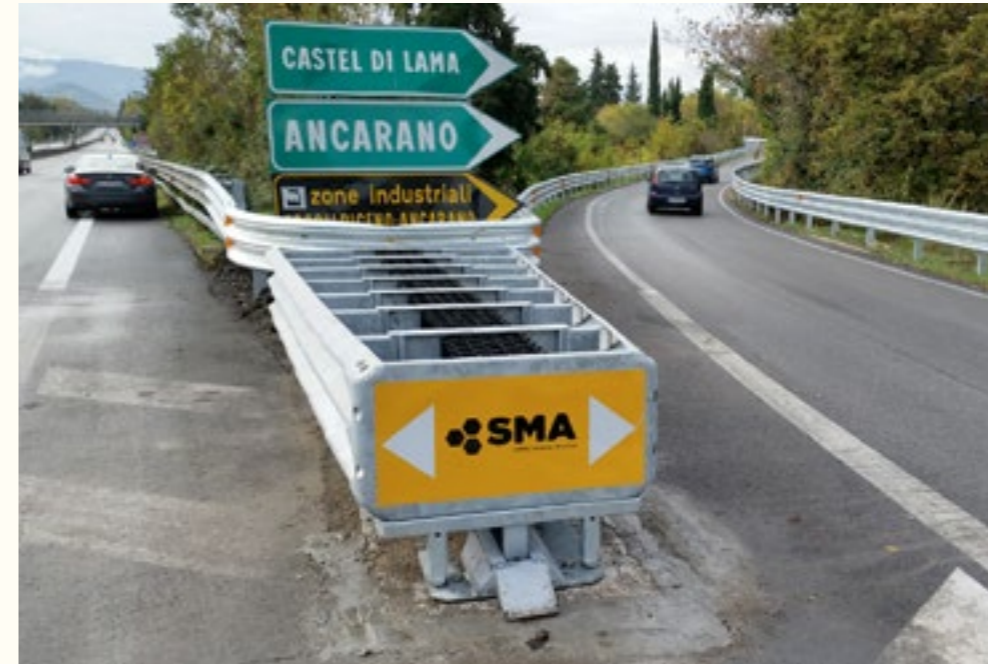
SMA 100W: installation on concrete basement
