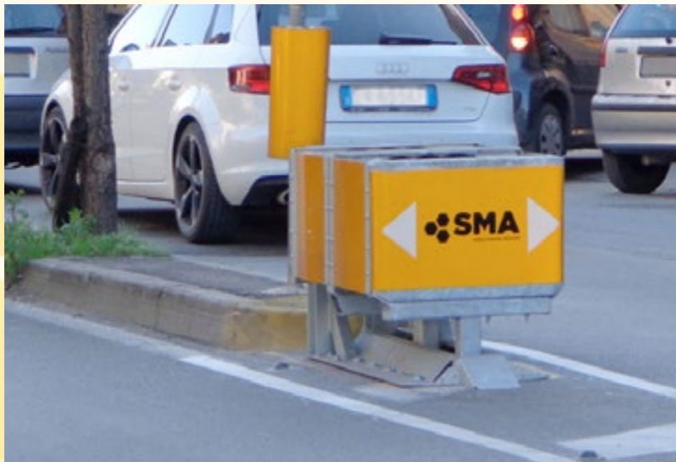
SMA City: installation on asphalt
