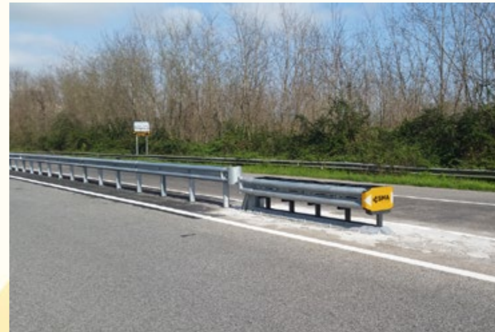
SMA A/T 80/1: installation on concrete basement
