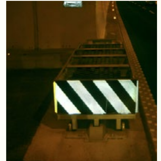
SMA 80P installed in the Frejus Road tunnel, Italy
