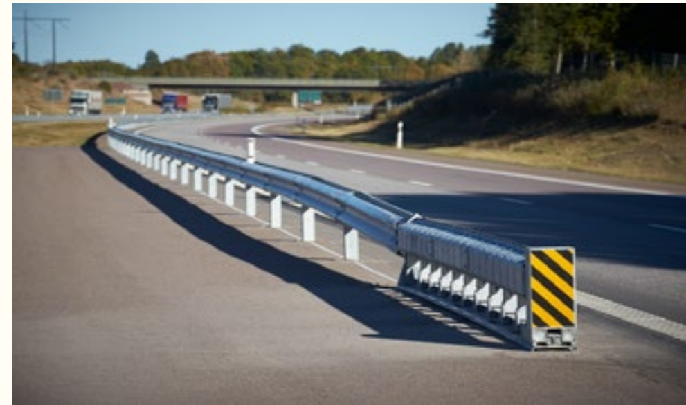
SMA T4: installation on asphalt
