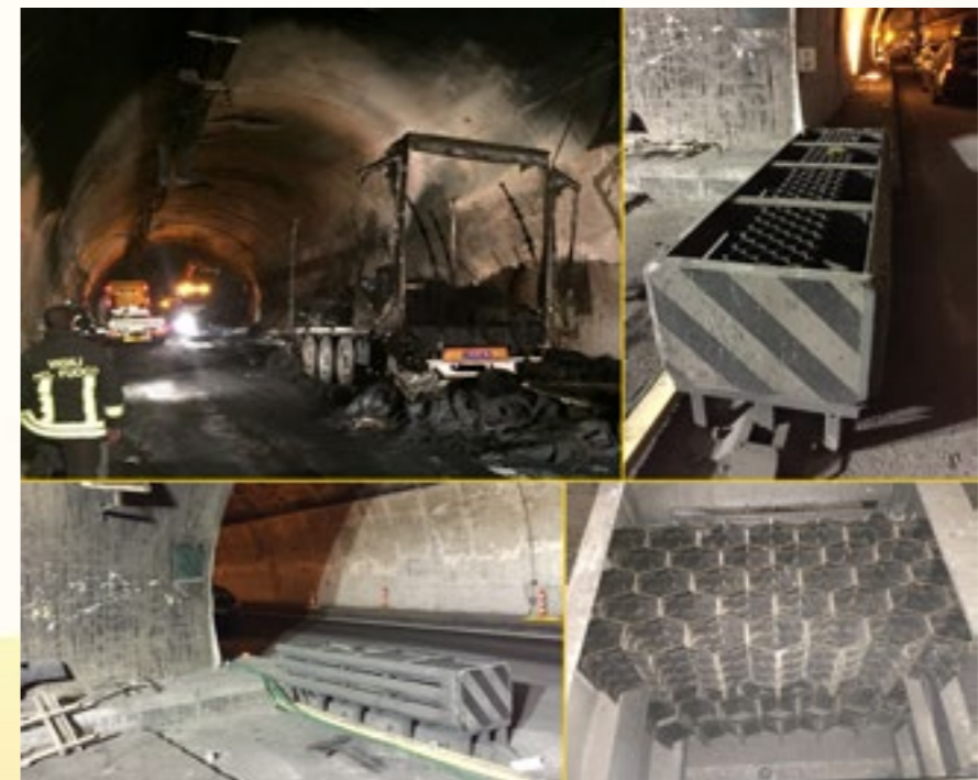
The pictures show the situation in a tunnel after a fire. The steel structure of the crash cushion has avoided the flame propagation.
