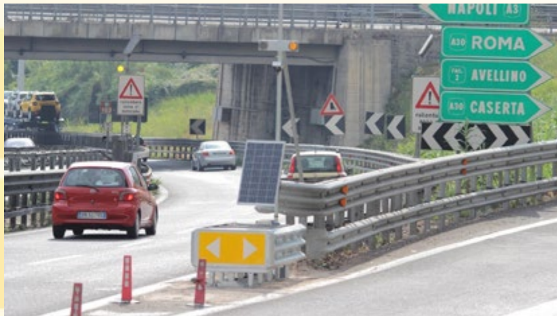
Example of a monitoring system GERONIMO installed on an Italian road. Click on the left picture to play the video.
